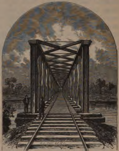
Bridge across the North Fork of the Canadian River, Indian Territory (M., K. & T. Railway).
